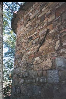
Catena metallica efficace.
