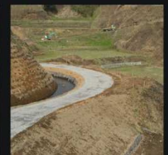
11 - after repaired 2.5m width pathway is constructing
