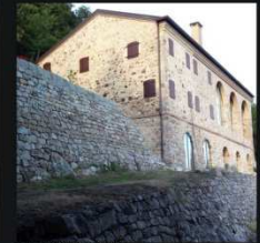
2 - rural house after restoration
