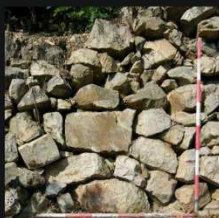
9 - front view of sections of dry-stone wall
