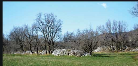
5 - In some areas it is hard to distinguish between dry stone walls, which divide the property, and slopes of the terraces
