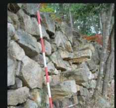
13 - side view of a section of dry-stone wall with corbelled steps
