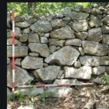
6 - front view of the retaining border wall
