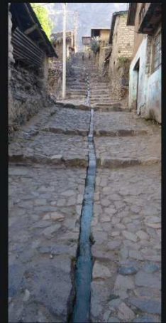
3 - a Laraos road, paved in stone with central water channel
