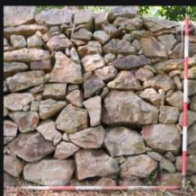
8 - front view of sections of dry-stone wall
