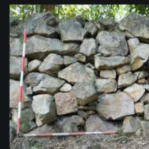
12 - front view of a section of dry-stone wall with corbelled steps
