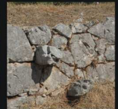
4 - protruding terrace stones making up steps
