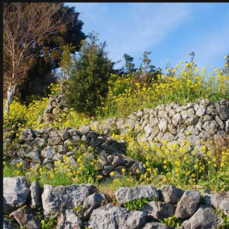
3 - dry stone wall of white limestone
