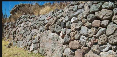
6 - detail of a wall rebuilt by the community of Soras
