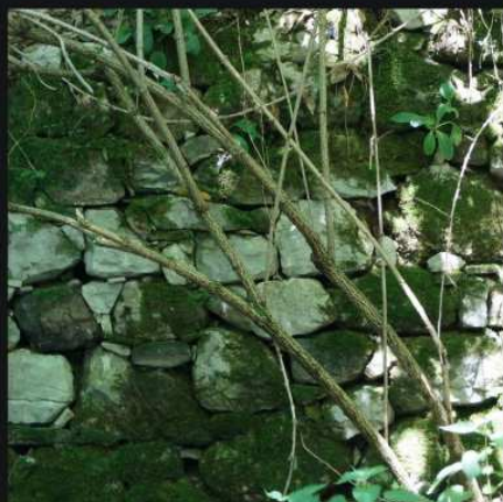
2 - the wall. Mountain longitudinal wall
