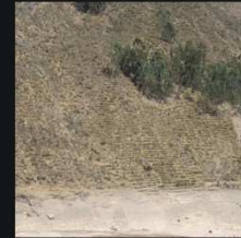
2 - slope of degraded and abandoned terraces - Cochupampa
