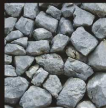
4 - detail of a dry stone wall
