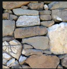
3 - detail of a dry wall
