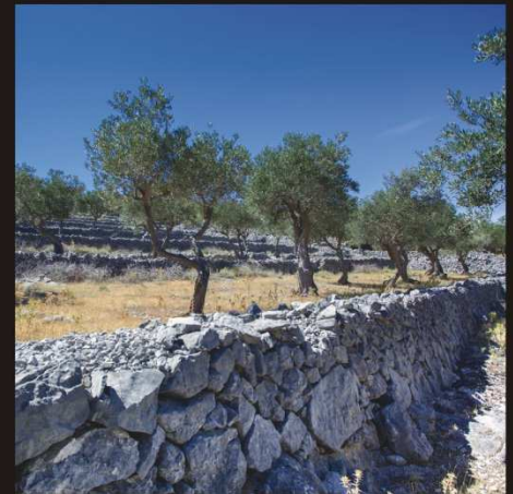
1 - terraces supported by dry stone walls
