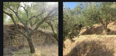
5 - dry sandstone walls marking the terracing of the olive grove
