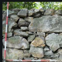
10 - front view of sections of dry-stone wall
