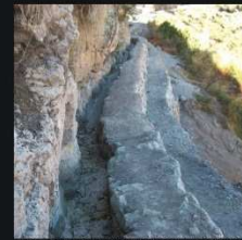
1 - detail of a diversion canal rebuilt by the community of Pampachiri
