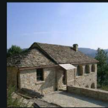
9 - Casera Piangrana the roof technique 'capra' returns
