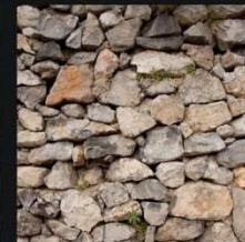
4 - Macerina drystone wall constructed without binders
