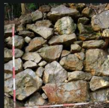
11 - front view of sections of dry-stone wall
